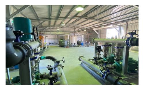
Recently, we added an additional ultra fine cartridge filter to support the four existing mineral media-based filters at the plant. These filters remove impurities and metals from the water sourced from the aquifer. Whilst the mineral media filters generally perform well, and the treated water meets ADWG<sup>1</sup> health requirements, we know from the feedback we receive that aesthetic qualities can be improved, such as reducing residual iron levels further.
